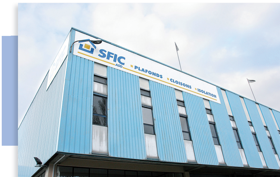
17, rue Montgolfier ROSNY-SOUS-BOIS (93) ▶
