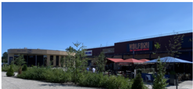
Chamblyrama - Facade restaurant Volfoni
